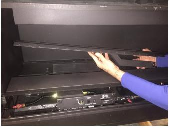
4. Use a ¼" nut driver to remove (4) screws (2/per side) securing the air shutter retainers (left and right) to the fireplace. Remove retainers to gain access to the burner orifices (set the retainers and screws aside for reinstallation).
