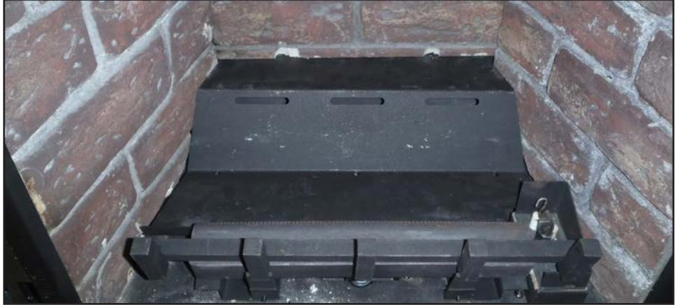
Figure 35. Empty firebox with grate and locator pins.
