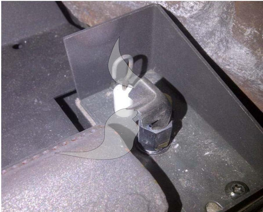
**Figure 24. Correct Burner & Pilot Shield Placement**
