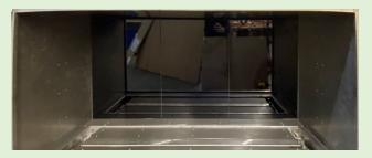
• Finally, install the left and right side firebacks (single-sided & see-through).
