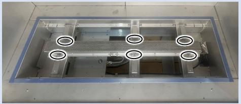
Use a 1/4" nut driver to remove the two screws that secure the pilot bracket to the right end of the burner. Carefully set the pilot assembly aside for reinstallation.
