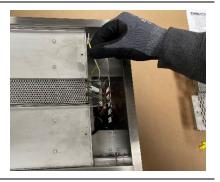
Route the wires from the 24VAC transformer through the strain relief at the bottom of the electrical box (below the pilot). Use listed low voltage wiring. Make sure to provide slack in the electrical line for removal and service.
