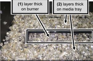
(b) Spread an even layer of crushed glass over the media tray and burner. The glass must be only (1) layer thick on the burner but can be (2) layers thick on the media tray. Excessive glass placed on the burner may cause poor burn characteristics and can lead to sooting and/or delayed ignitions.
