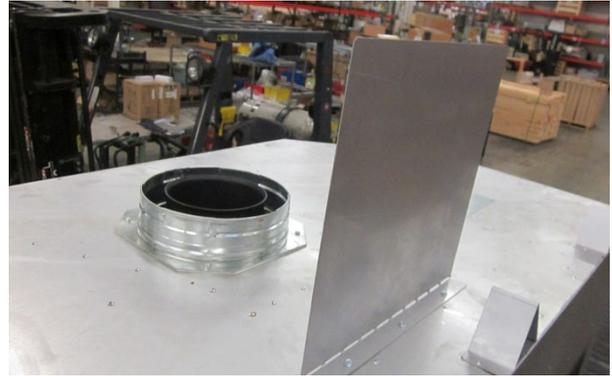
**Horizontal Terminations Require Vinyl Standoff and Termination Shield (on Combustible walls only)**
