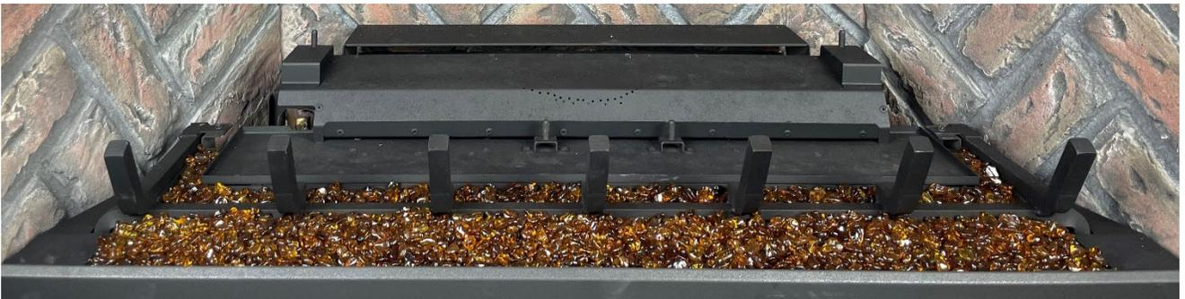
2. Lightly dress the ember glass with black touch-up paint (we recommend Stove Bright®). Check the appearance with the lights on and add additional paint, as needed, for a realistic glowing ember appearance.
