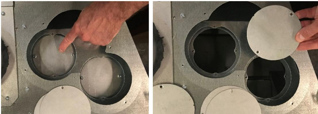
4. Remove the left, top layer, cover plate. Turn it over and then reinstall it in place of the right cover plate removed in step 1. Replace all screws so there are no holes left in the top of the fireplace.
