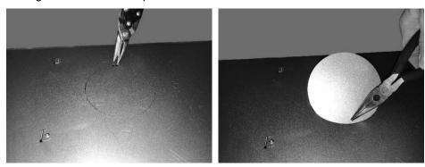
Grab on to the knockout with pliers and bend it back and forth until the remaining tabs break free. Discard the knock out plate.
