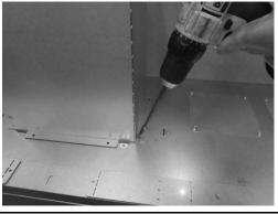
The (2) header standoffs are screwed down flat to the front edge of the top of the fireplace. On each standoff, remove the screw that is closest to the center of the fireplace. Bend the legs at the perforations as shown below and attach the foot of the standoff to the top of the fireplace using the screw removed earlier in this step.
