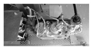
7. Make the gas line connection, bleed the gas line (if applicable), start the heater and thoroughly leak-test all gas connections and the gas control valve.
