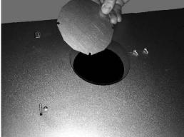
Insert a starter collar into each of the holes that were uncovered in the previous step and bend the tabs to secure the starter collar to the fireplace.. Seal the joints with silicone caulk or aluminum (U.L. 181A-P) tape
