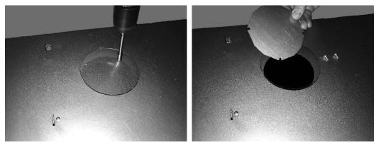
5 Install the Convection Air Deflectors. The (2) deflectors must be installed prior to attaching the CoolSmart kit. After removing the cover plates, install the deflectors as shown below.
