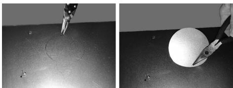
3 Grab on to the knockout with pliers and bend it back and forth until the remaining tabs break free. Discard the knock out plate.
