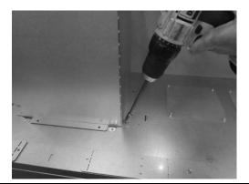
3 The (2) header standoffs are screwed down flat to front edge of the top of the fireplace. On each standoff, remove the screw that is closest to the center of the fireplace (keep screw for reinstallation). Bend the legs at the perforations as shown below and attach the foot of the standoff to the top of the fireplace using the screw removed earlier in this step.
