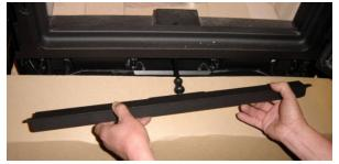
Install the ash guard as shown below. Note how the horizontal tab fits in front of the door opening.
