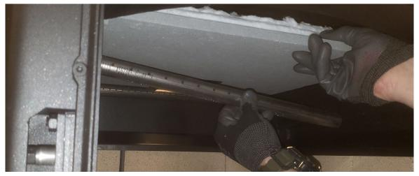
7 Gently slide the baffle board and blanket forward until it is free of the rear air tube. Lower the front edge of the baffle and fold the edges of the blanket inward.
