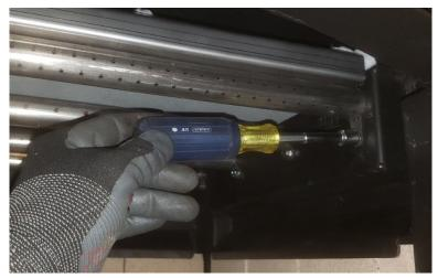
Push up on the baffle slightly and slide the front air tube to the left until the end is clear of the manifold. Lower the right end of the tube and maneuver left end of the tube out of the manifold on the left side of the firebox.
