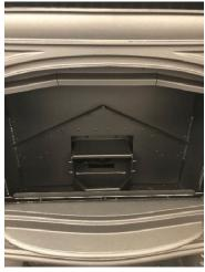
8. With the liners removed, clean all fly ash and debris from the firebox. Clean the liners before replacing them. Make sure to clean the heat exchanger on the firebox ceiling.
