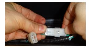
3 Remove the assembly by slightly lifting the right side and slide it to the right. This will disengage the main connector from the valve. Once the Electronic Controls Assembly is disconnected from the valve, slide it forward, out of the appliance. The pilot wires will still be connected and are long enough allow the assembly to be pulled clear of the unit. Make sure to not damage the pilot wires.
