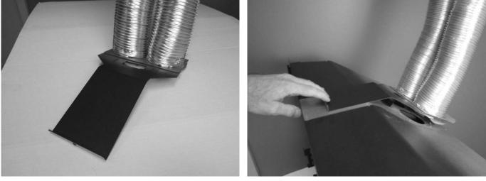
Secure the vent connector to the insert using the screw removed earlier.
