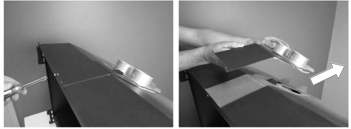
Connect the flex vent (exhaust and intake) to the vent connector (use self-drilling screws or hose clamps).
