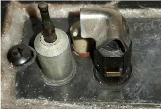
**Figure 29 – Pilot in LP (slide gate to rear of Pilot Tower)**
